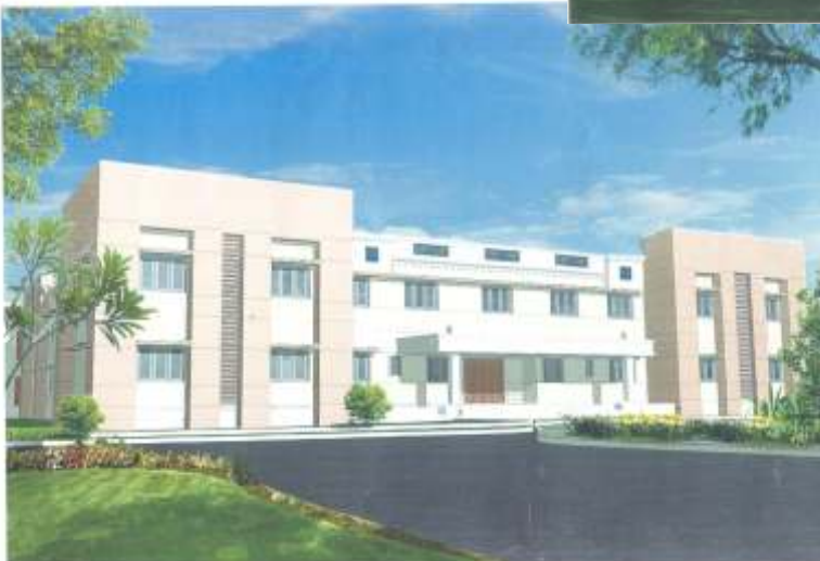
Proposed Ladies Hostel with 84 Rooms. This Building is partly financed by UGC.
